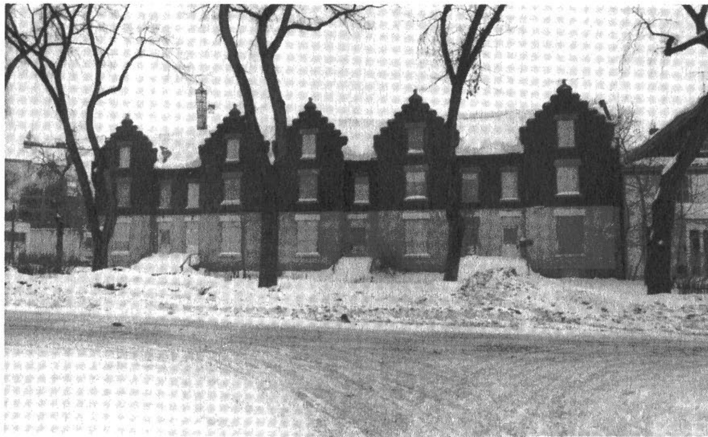
281-289 Spence Street, vacant and boarded up-1979.
