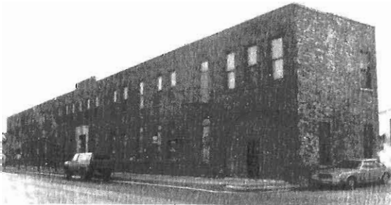
The former station building, 1982. The bricked-in archway is visible at the lane.
