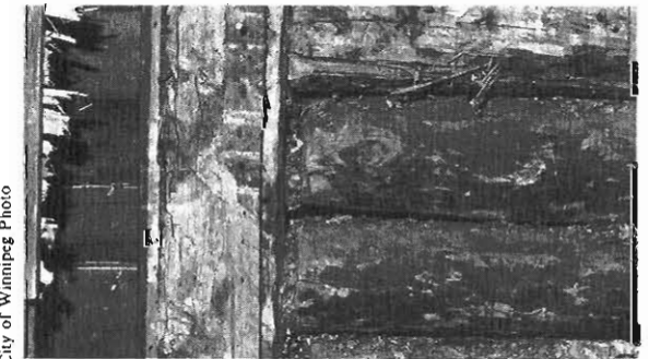
Wall detail showing a modified “Red River Frame” style of log construction.
