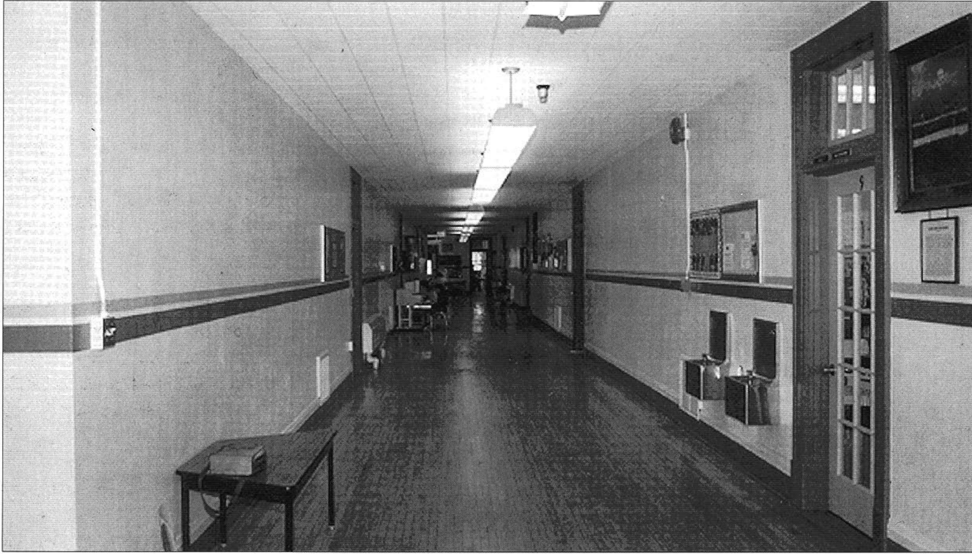
An interior hallway. City of Winnipeg
