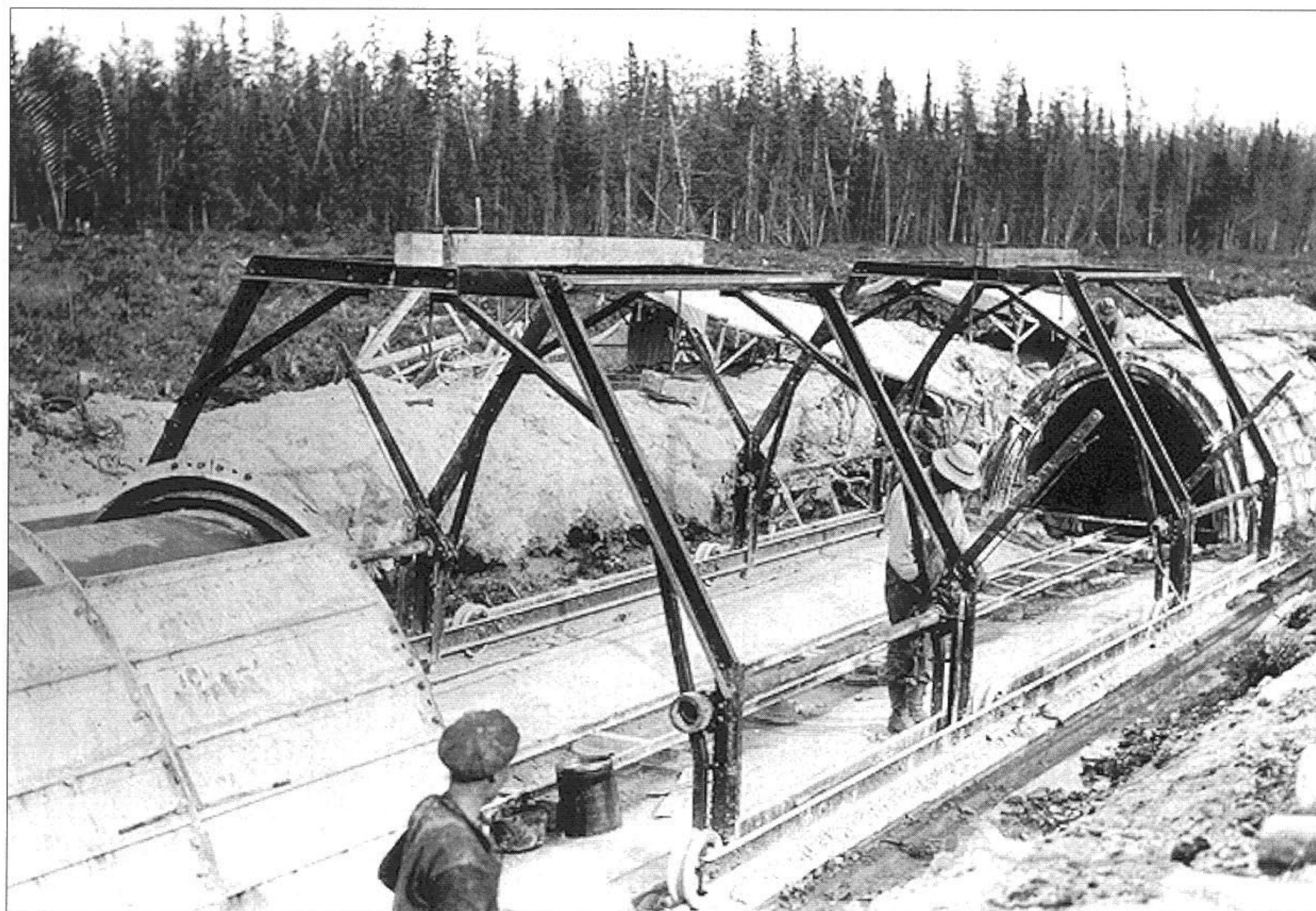
Construction of the aqueduct, c.1917. Western Canada Pictorial Index
