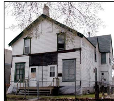
John Villiers Duplex, 332-334 Ross Avenue
