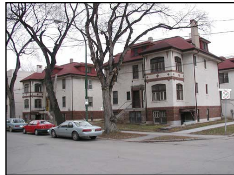
Two of the eight separate buildings that make up the Chelsea Court Apartments, 440-442 Assiniboine Avenue
