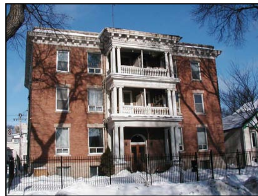
Ludlow Court Apartments, 141 River Avenue with its imposing front porch
