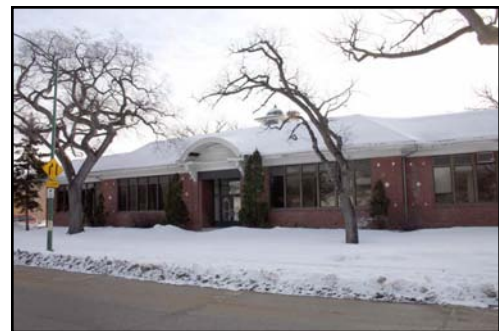
Main (west) façade of Anna Gibson School, 77 Henderson Highway, shortly before its demolition
