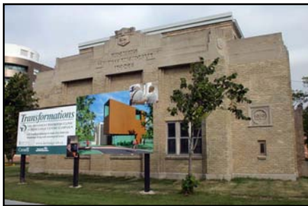
Sign announcing renovations and alterations in front of the Women's Tribute Memorial Lodge, 200 Woodlawn Street
