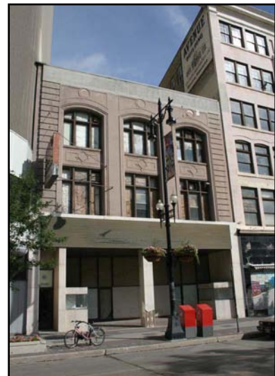
Hample Building, 271 Portage Avenue
