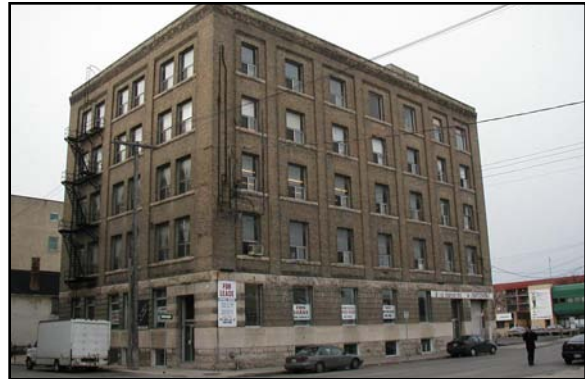
The main façades (north and east) of the Former Henderson Building, 332 Bannatyne Avenue
