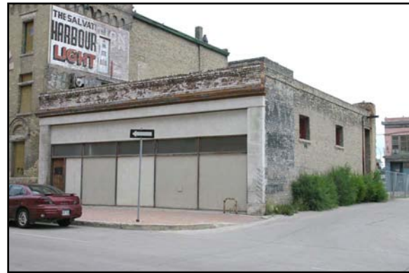
Small retail block, 217 Rupert Avenue shortly before demolition
