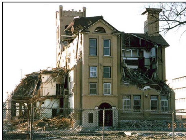
Demolition of the J.B. Somerset (Sacre-Coeur School No. 2), March 2005
