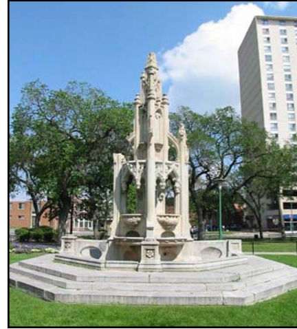
The damaged Waddell Fountain, Central Park
