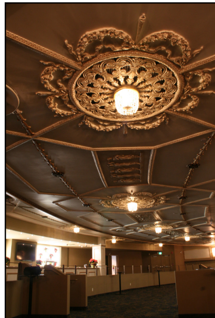
Renovated interior of the Metropolitan Theatre, 281 Donald Street
