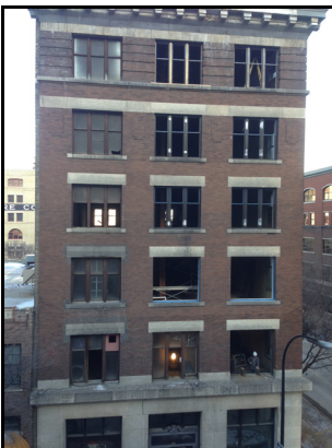
165 McDermot Avenue, window replacement, 2014
