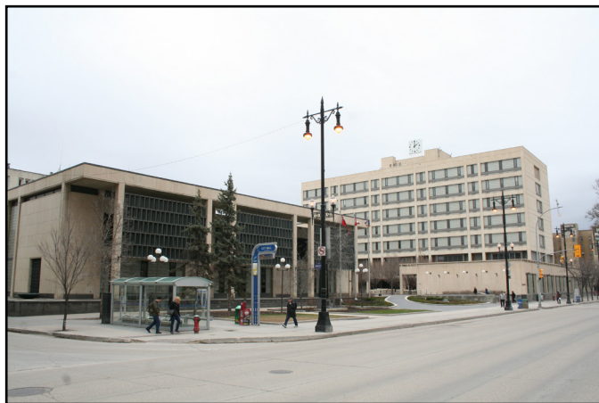
Winnipeg's City Hall complex
