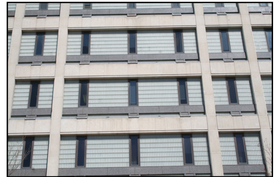
Detail of the south façade of the Administrative Building
