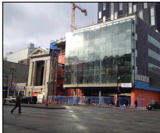
2014 construction of Centrepoint
