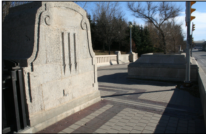
Stone ornamentation on the Main Street Bridge
