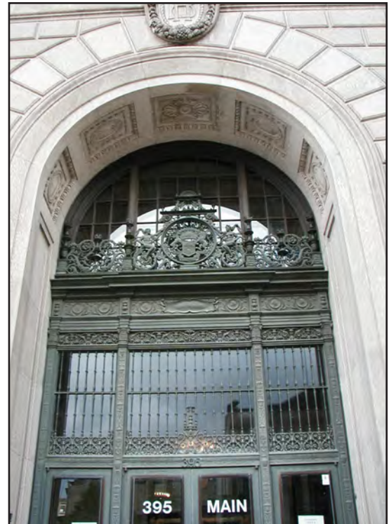
Bank of Hamilton, 395 Main Street, detail of main doors, 2004
