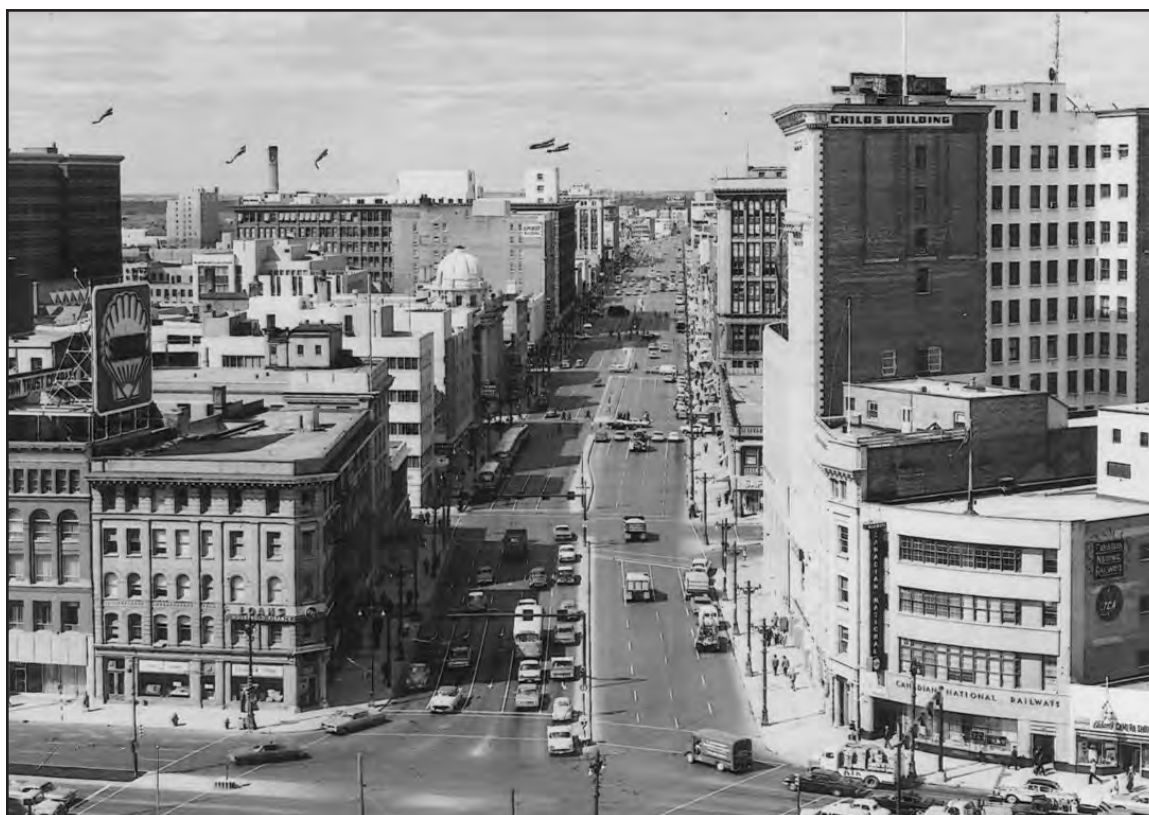
Looking west down Portage Avenue from Main Street
