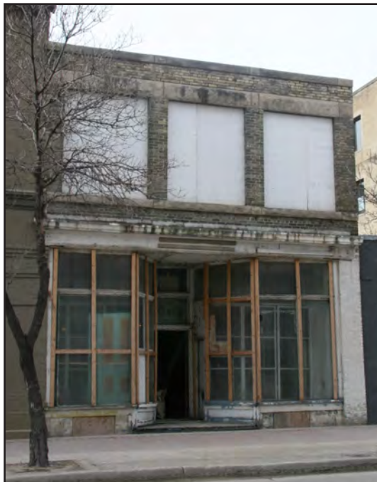
Winnipeg Saddlery Building, 284 William Avenue, main façade, 2015
