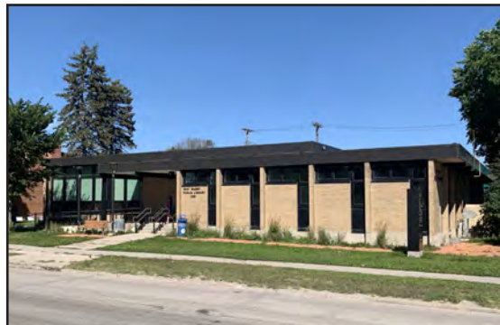
Fort Garry Public Library, 1360 Pembina Highway, 2022, Nominated List
