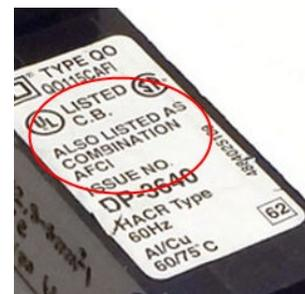
Sample Labels on Combination-Type AFCI Breakers
