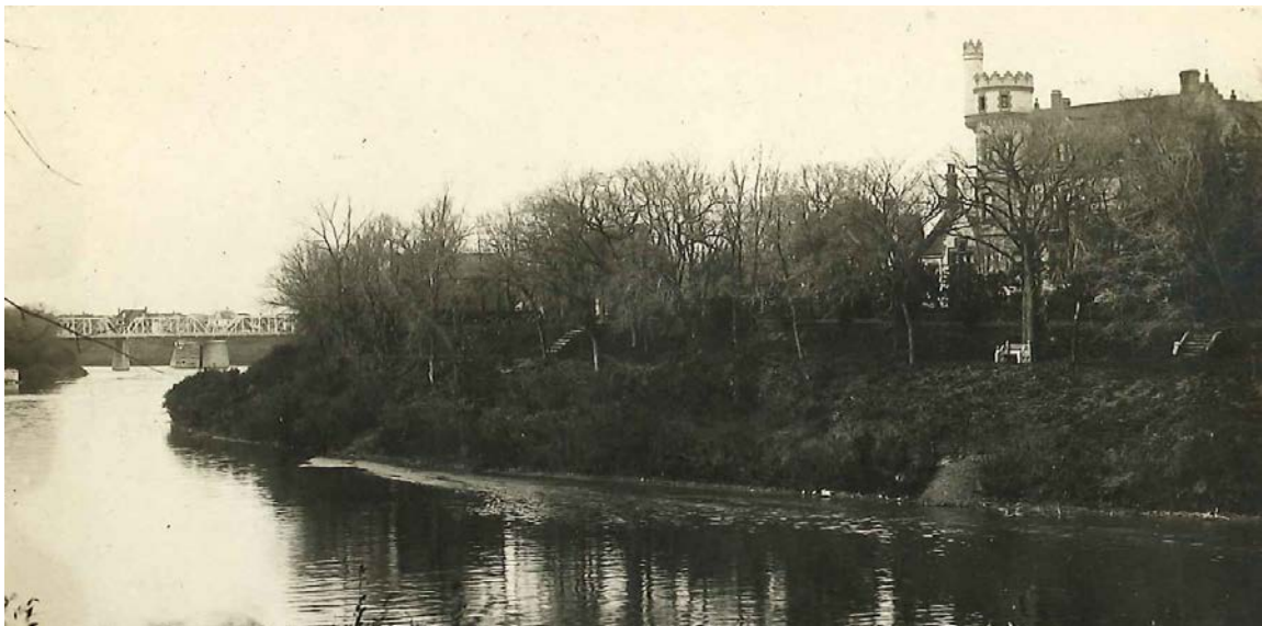
Historic Photo of Armstrong's Point and the Maryland Bridge
