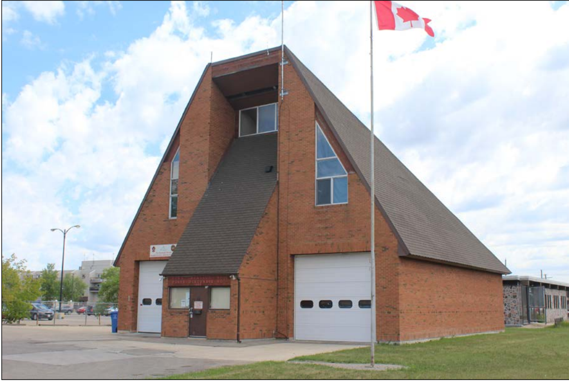
Plate 27 – Fire Hall No. 15, 1083 Autumnwood Drive, front (west) and south façades, 2021. ( M. Peterson, 2021. )
