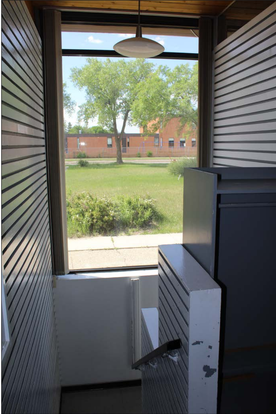
Plate 25 – Windsor Park Library Branch, 955 Cottonwood Road, southeast staircase, 2021. ( M. Peterson, 2021. )
