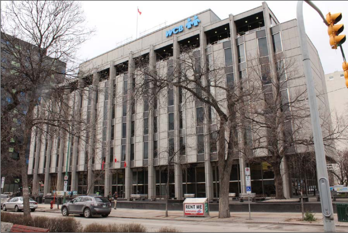
Plate 6 – Monarch Life Building, 333 Broadway, south façade, built 1961, 2016. ( M. Peterson, 2016. )
