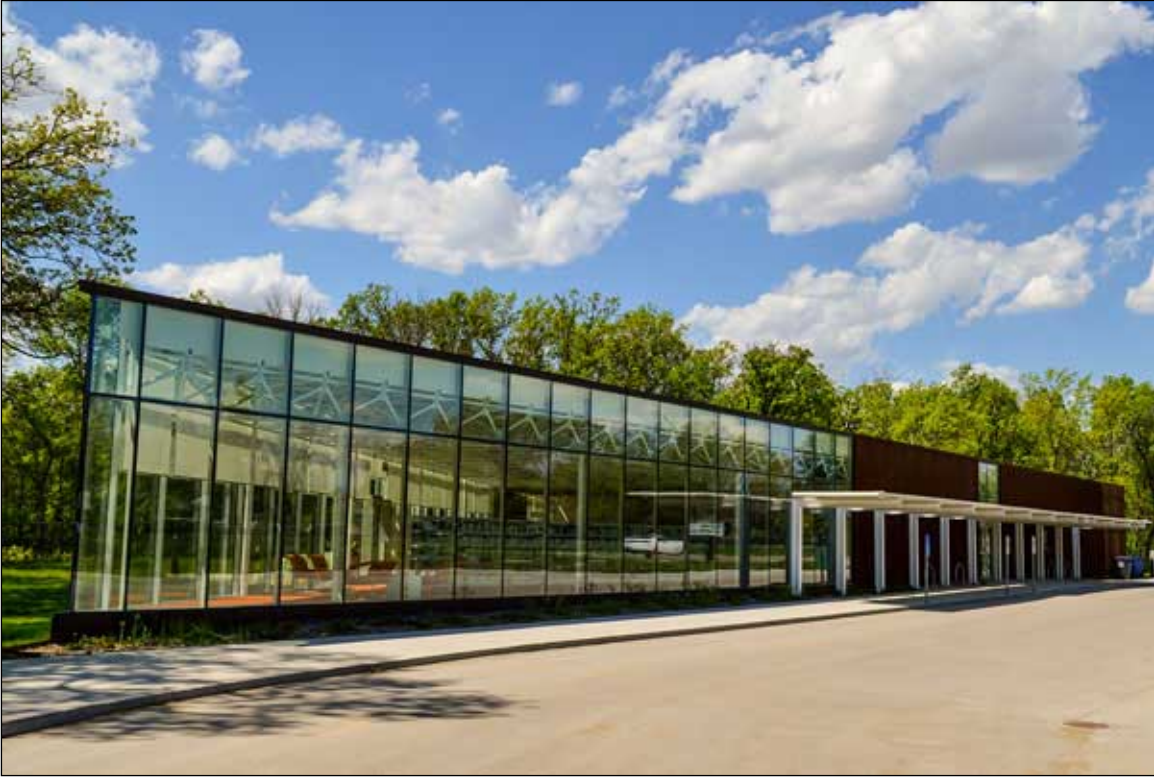
Plate 30 – Windsor Park Library, 1195 Archibald St., ca.2018 ( City of Winnipeg, Libraries Branch. )
