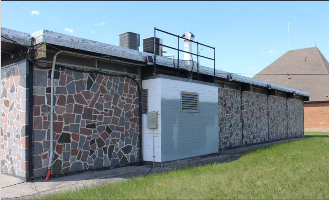
Plate 17 – Windsor Park Library Branch, 955 Cottonwood Road, rear (north) façade, 2021. ( M. Peterson, 2021. )
