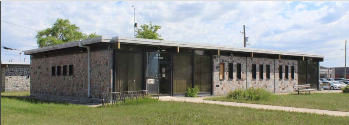
Plate 13 – Windsor Park Library Branch, 955 Cottonwood Road, front (south) and west façades, 2021. ( M. Peterson, 2021. )
