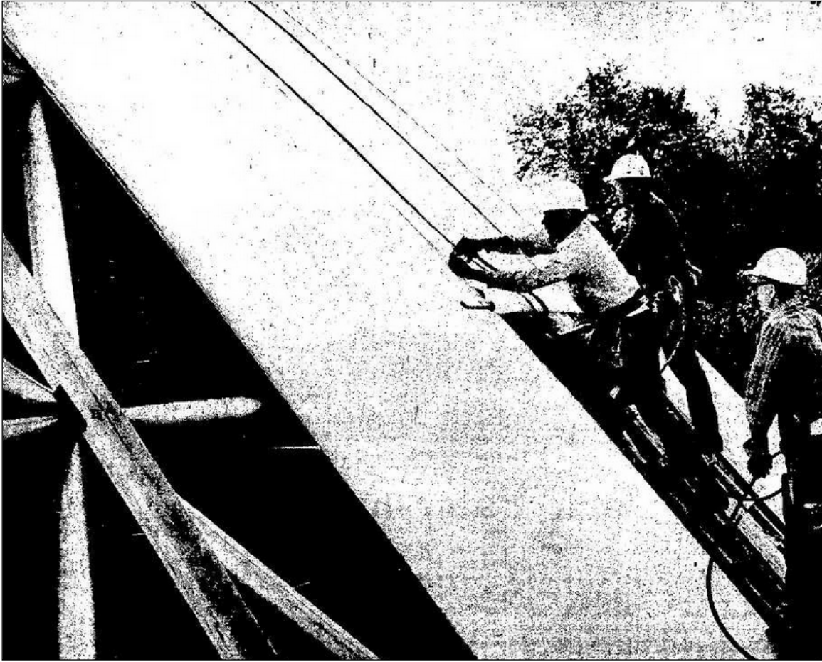
Plate 34 – Affixing the roofing material to the domed roof ribbing of Rainbow Stage. ( Winnipeg Free Press, July 25, 1970, p. 5. )
