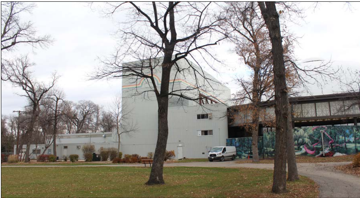
Plate 47 – West side of rear of Rainbow Stage, Kildonan Park, 2015 Main Street, 2022. ( M. Peterson, 2022. )
