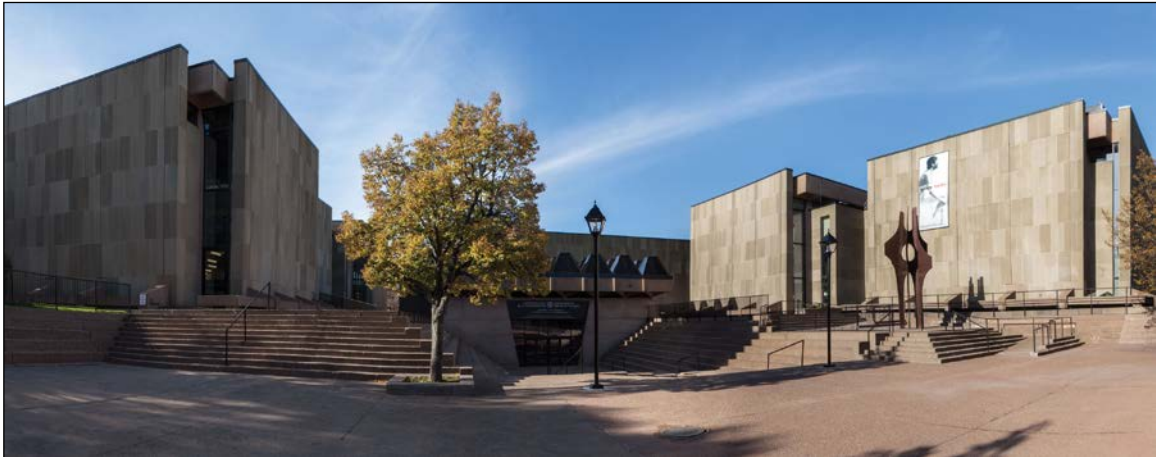
Plate 20 – Confederation Centre of the Arts, Charlottetown, P.E.I., opened in 1964, designated a National Historic Site in 2003 because, according to the Historic Sites and Monuments Board of Canada, “it is a distinguished example of Brutalist architecture in Canada.” (Photograph by Centre des arts de la Confédération, World Architecture website, no date.)
