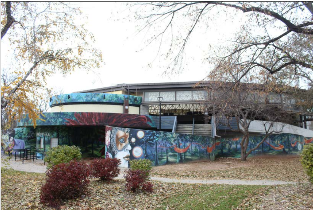
Plate 40 – Main entrance, south side, Rainbow Stage, Kildonan Park, 2015 Main Street, 2022. ( M. Peterson, 2022. )
