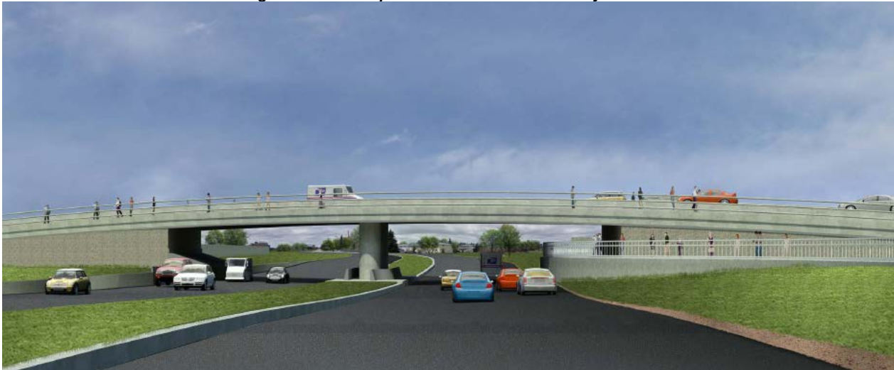
Figure 1: Grade Separation Structure at Rothesay Street
