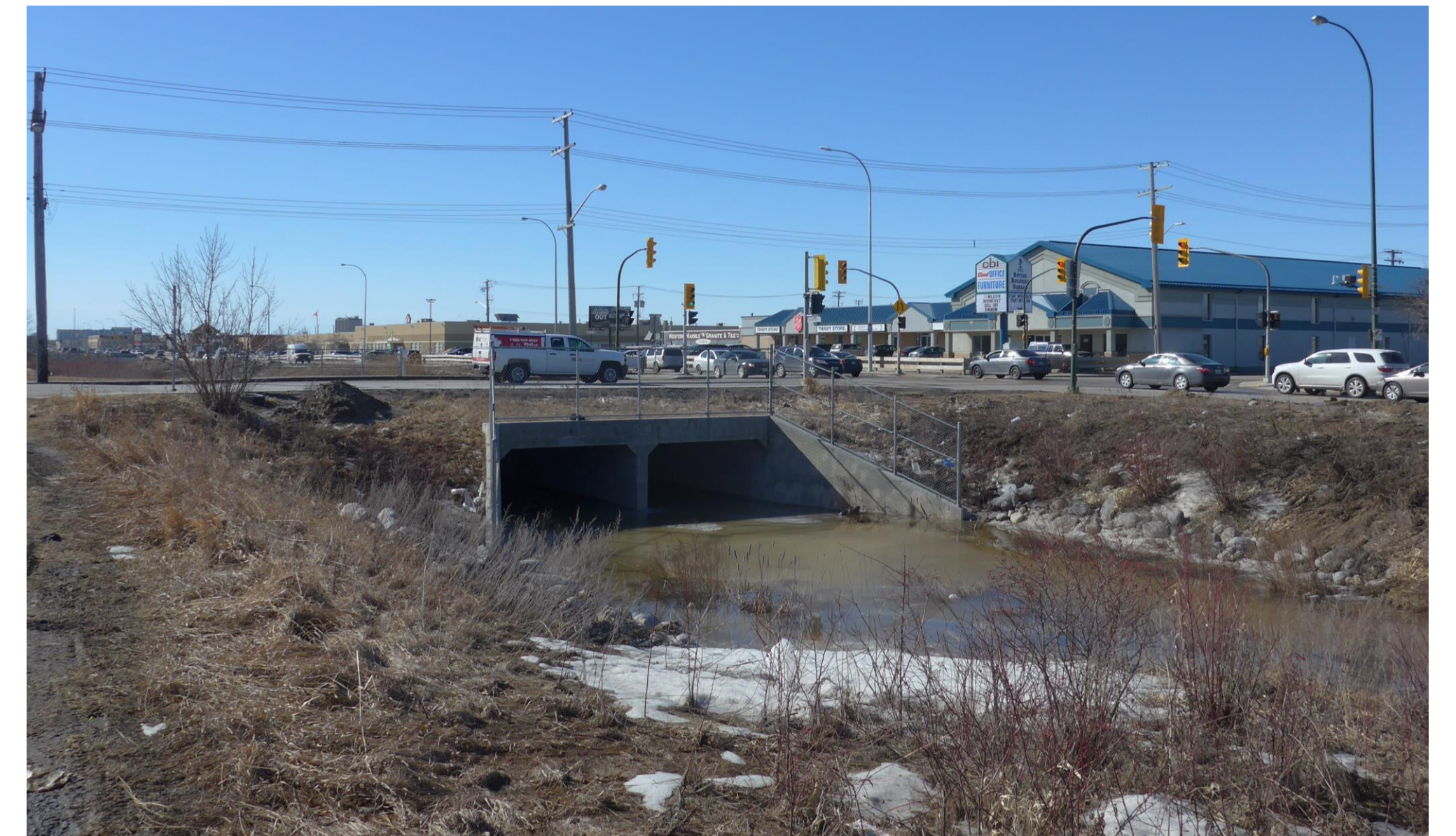
Example of an existing culvert in Winnipeg that is similarly shaped as the proposed culvert at Rue des Trappistes over Westendorf Coulee.
