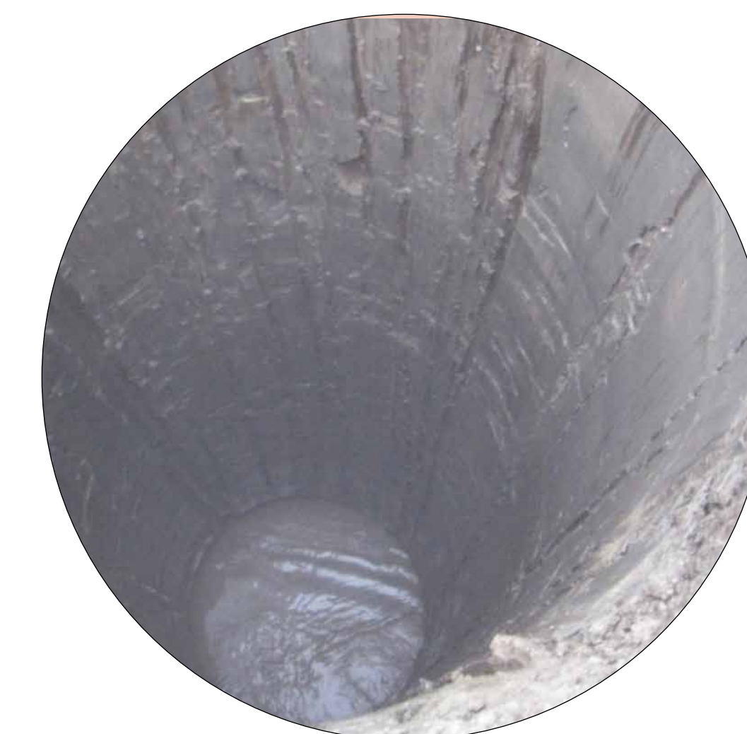
Completed drilled shaft.
