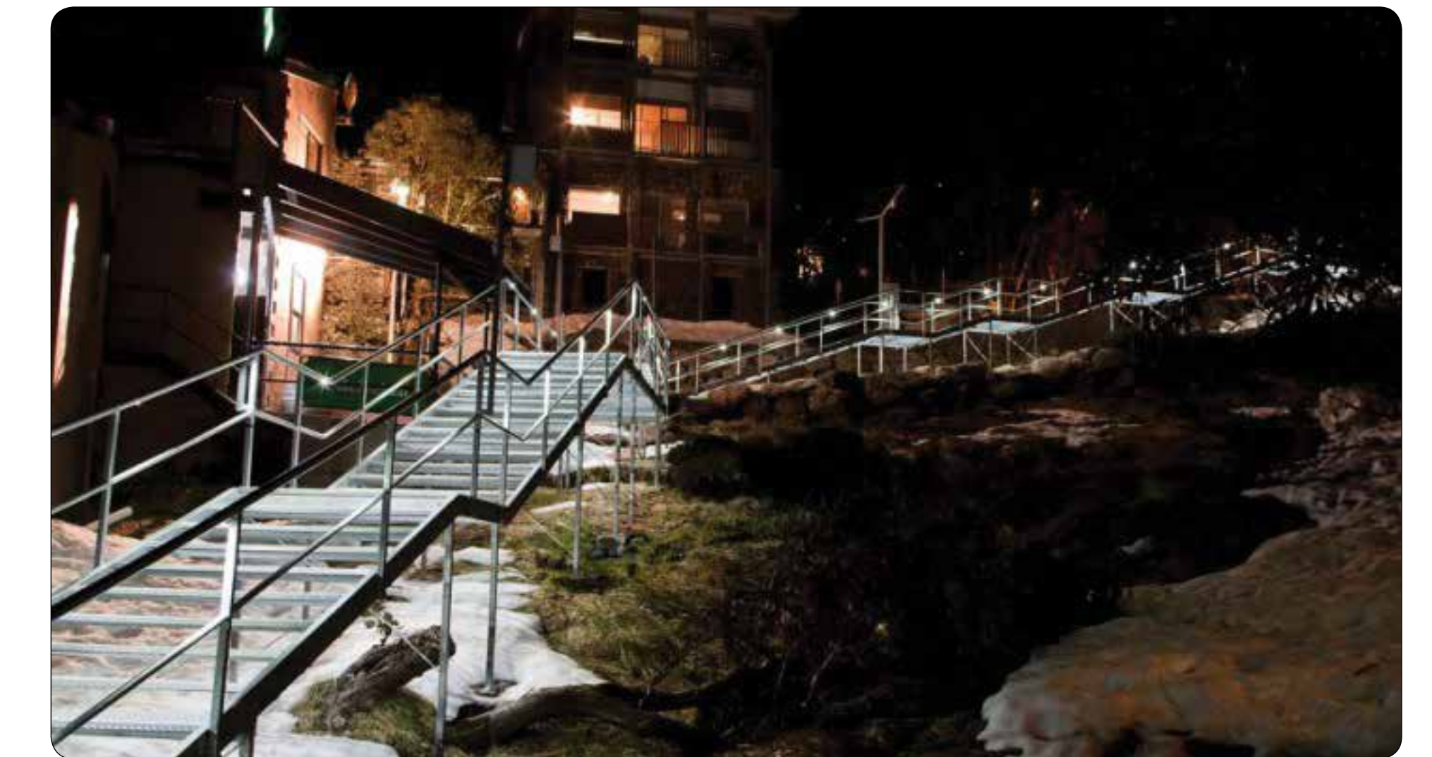
LED handrail lighting example
