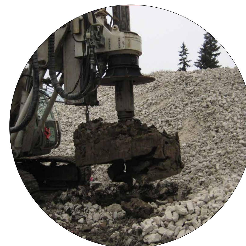
Large auger used to drill holes for rockfill columns
