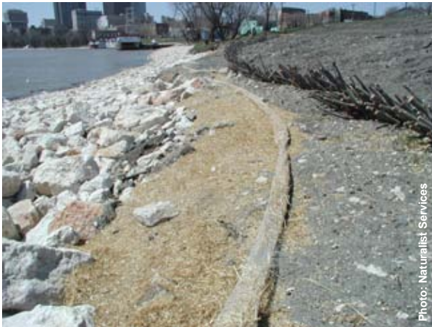
Willow Posts – at installation
