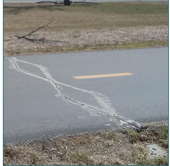
Figure 1: Inductive loop sensor for counting bikes
