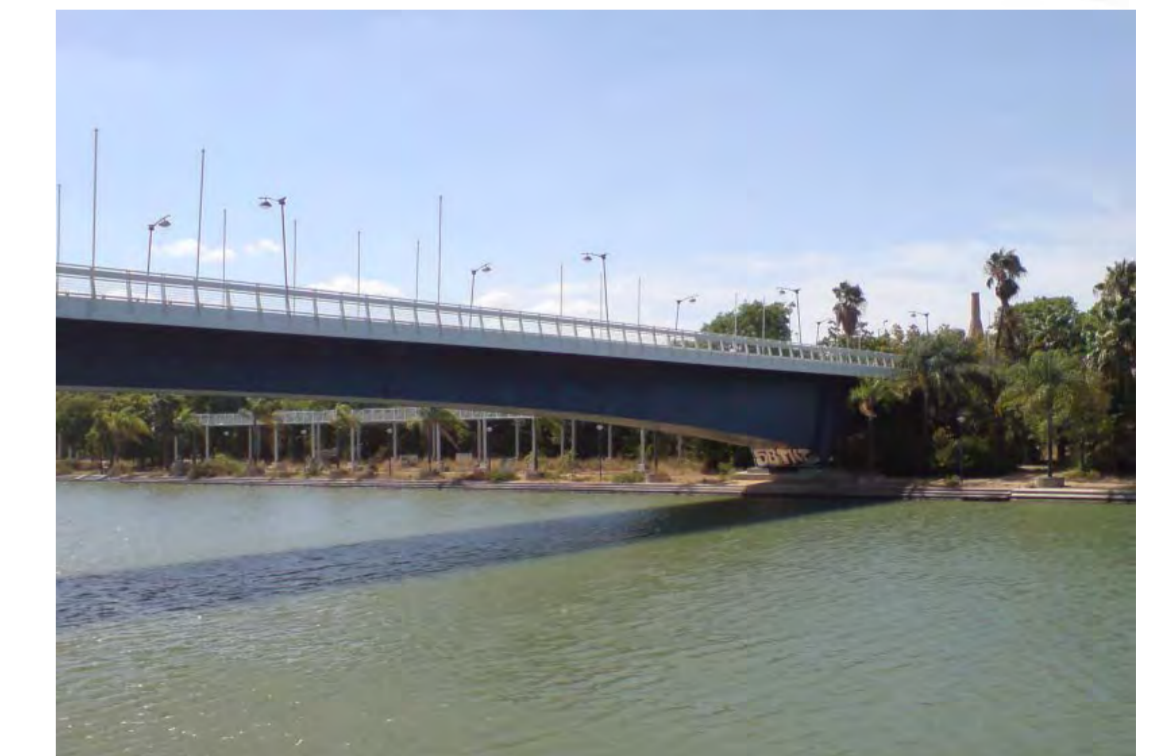
Example of existing girder bridge
