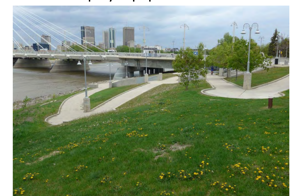
New accessible ramp to river
