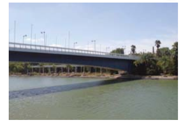
Example of existing girder bridge
