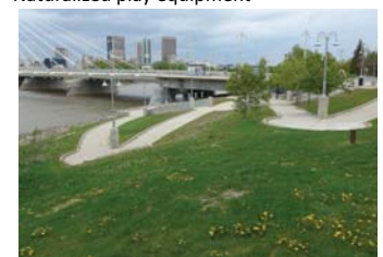
New accessible ramp to river
