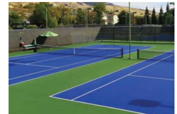
Upgrade tennis court
