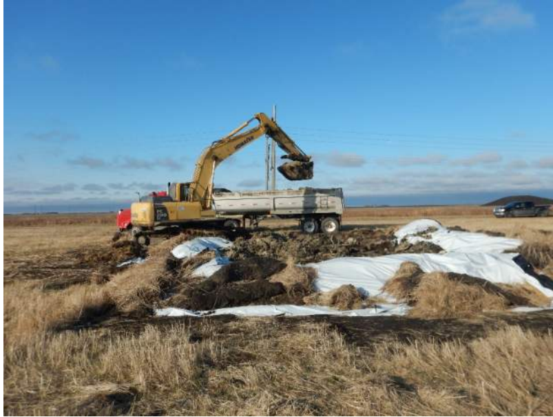
Photograph 3. Decommissioning of Biosolids Pilot Odour Assessment - Plot 5, Removal of Biosolids.
