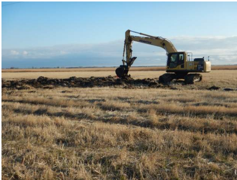
Photograph 4. Decommissioning of Biosolids Pilot Odour Assessment - Plot 7, Levelling of Clay Berm.
