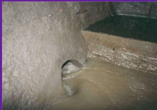
Images from inside the trunk sewer near the outfall; left image shows the weir and flap gate with water trapped in between; right image shows the weir and off-take pipe that diverts dry weather flows to treatment, note the difference in sizes between the off-take and trunk sewer
