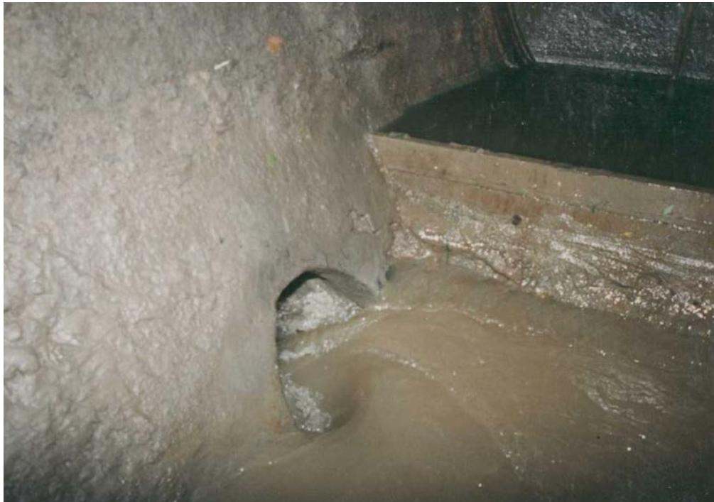
Figure 7-6. Typical Combined Sewer Diversion Weir and Off-take Pipe
