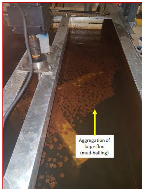
Figure 5-18: Aggregation of large floc (mud-balling effect) in DAF Tank #3
