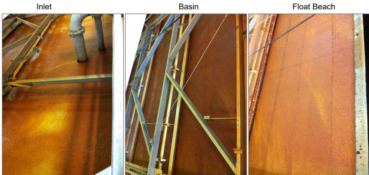
Figure 2-4: Visual inspection of a DAF basin top.
